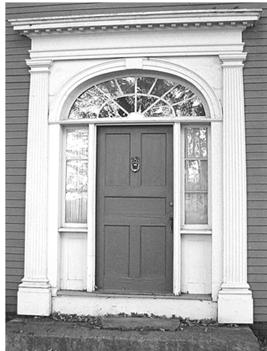
Built in 1831 by George West, Esq., the Hall House is one of the finest examples of Federal Style architecture in Orleans County. The front entry, shown above, is graced by side and fan lights set within Doric pilasters. Inside, an ample hallway with open stairs gives access to two nicely proportioned parlors, an office with separate side entrance, a large kitchen with pantry, and a bath. The first floor features nine-foot ceilings and four fireplaces. The trim in the north parlor shows Greek Revival influence. The second floor contains three large and two small bedrooms.
